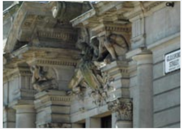
▲Glasgow is well known for its beautifully preserved Georgian Architecture that can be seen all over the city
